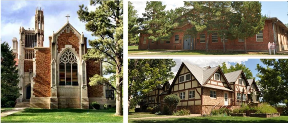
Historic buildings in the monastery campus area are aesthetically striking and structurally sound, creating an opportunity for historic preservation. Clockwise from left: the monastery and chapel, the fieldhouse, and the Sister’s House. Images courtesy The Abbey Events Complex.
